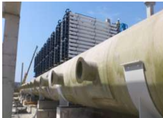
Erection of RO Plant – November 2012
